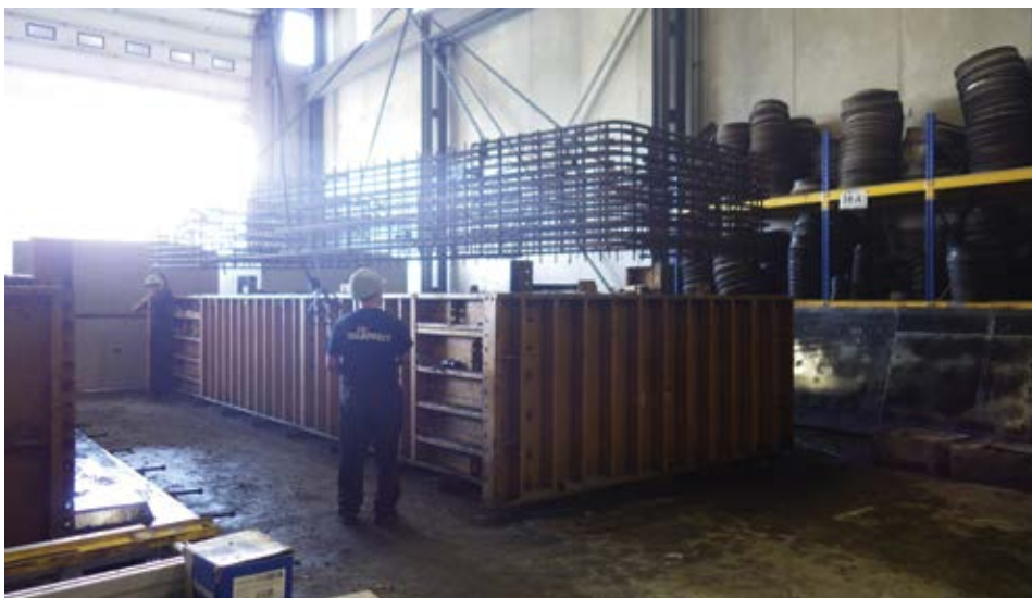
Pre-welded cage being lowered into the mold jacket
