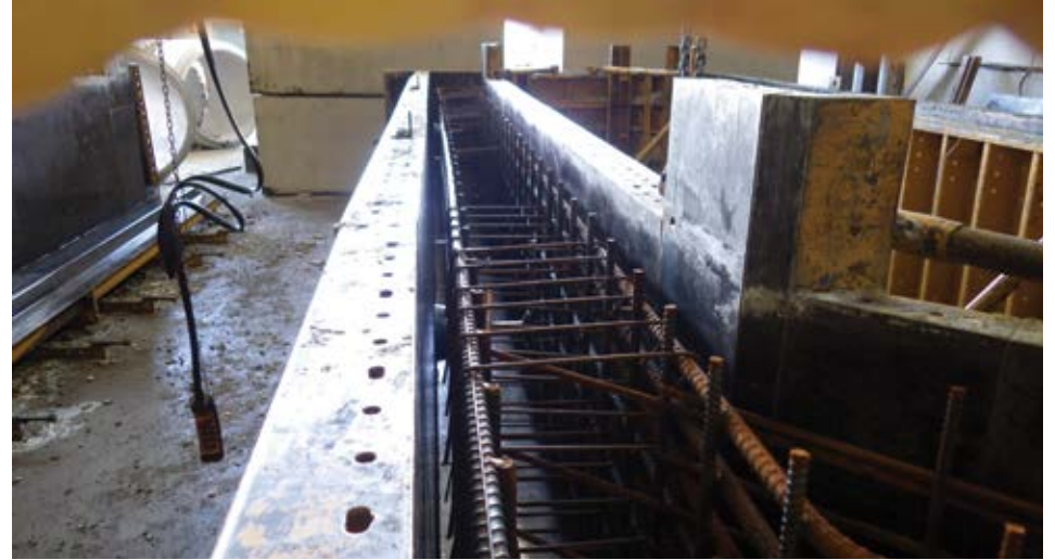
Cage placed into the form in preparation to receive concrete
