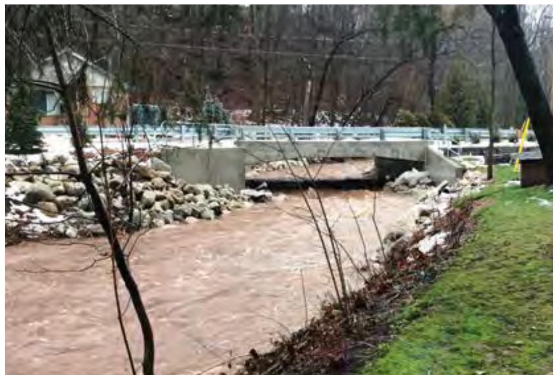
Completed Bridge in Service
