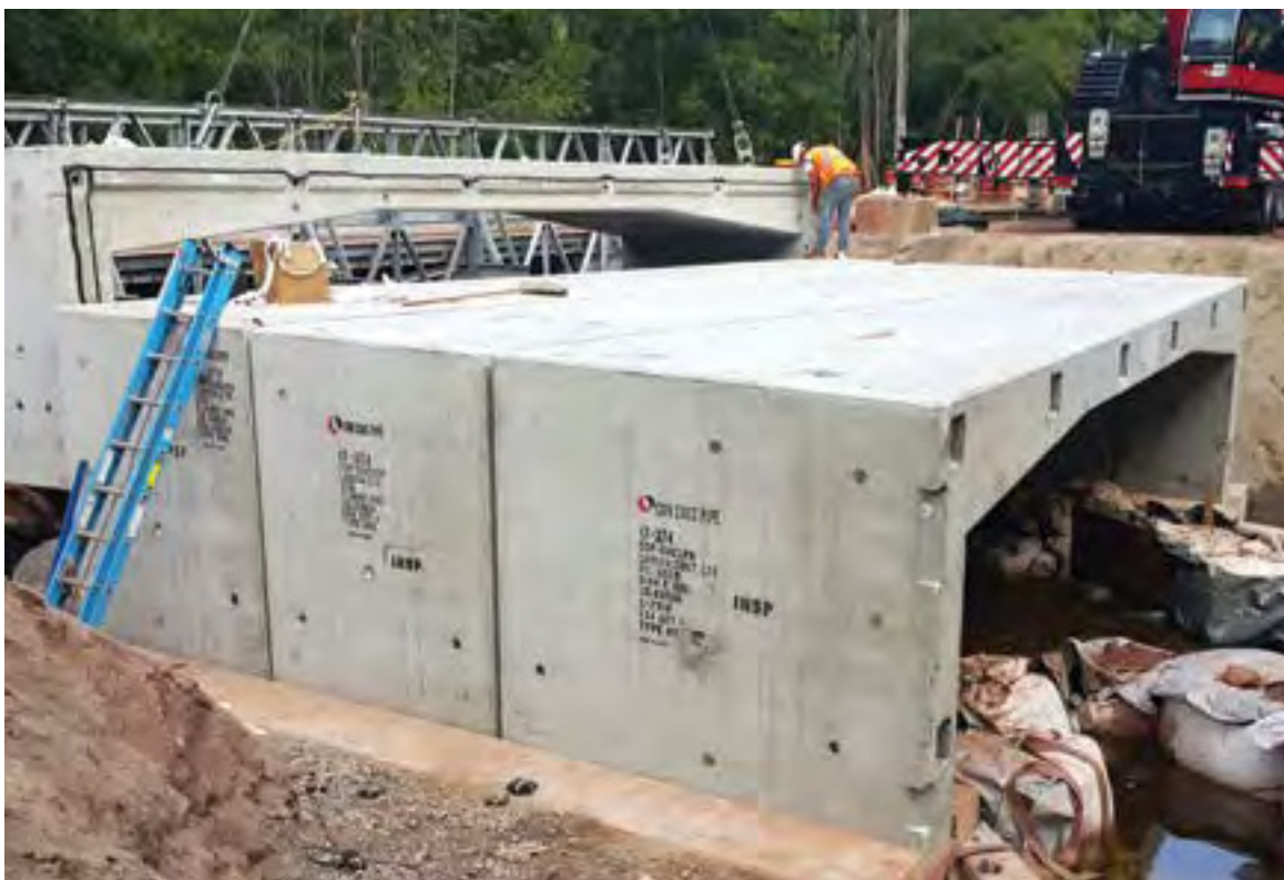
Three-sided precast box units being installed
